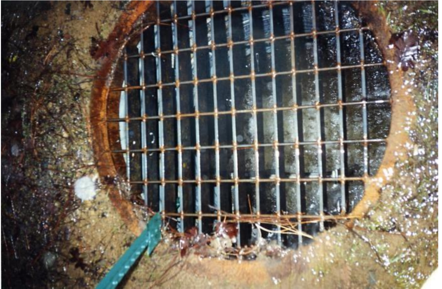
THE SURFACE DRAIN
