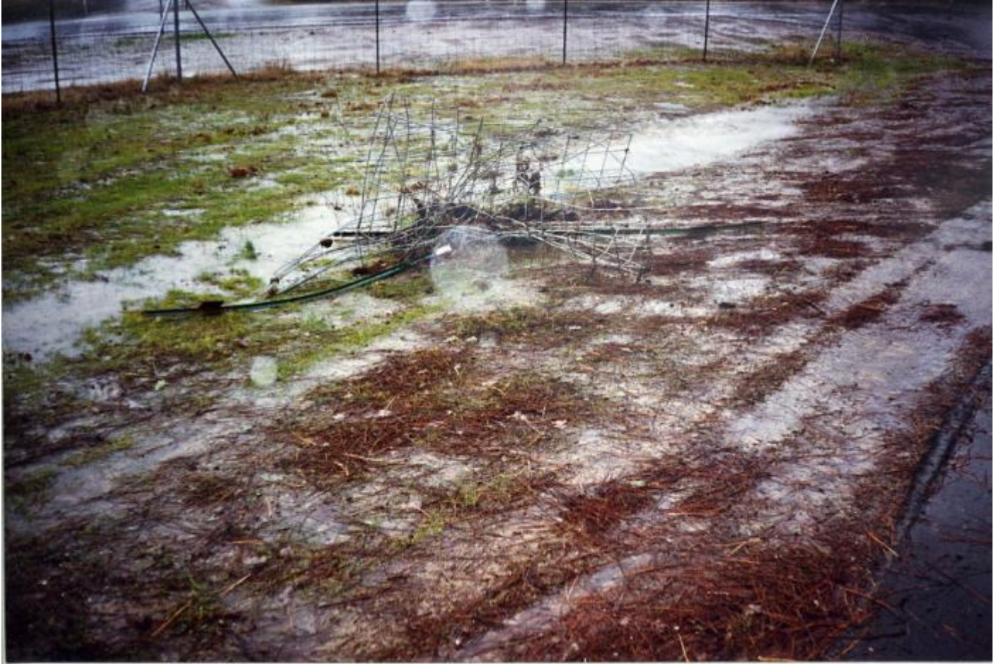
THE BLOCKAGE REMOVED
